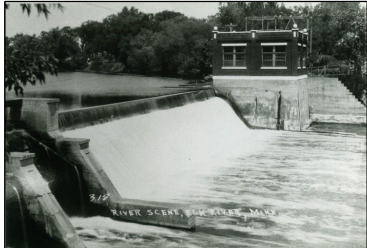
Postcard view of dam and power plant, ca. 1920 (Lyle Collins Collection)
