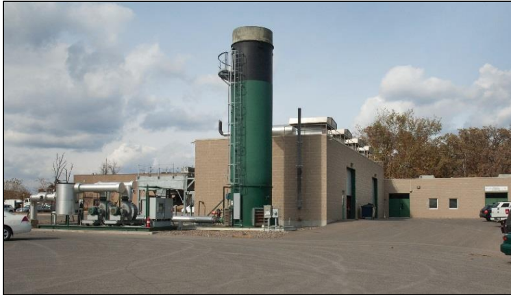
Electric Generation Facility at the Elk River Landfill (Elk River Municipal Utilities)
