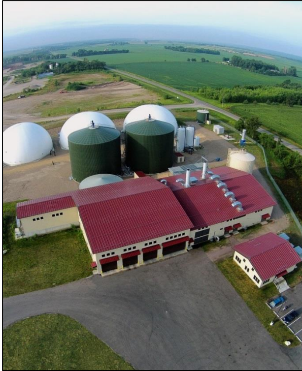
Hometown BioEnergy Facility in Le Sueur, Minnesota (Avant Energy)
