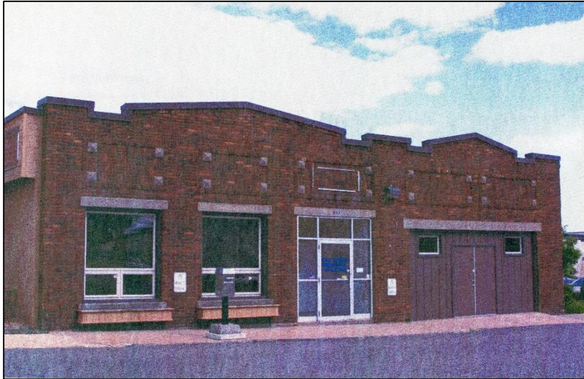
Former ERMU Office at 322 King Avenue (Elk River Municipal Utilities)
