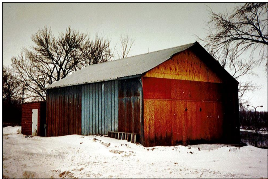
Storage Building by the Old Creamery (Elk River Municipal Utilities)
