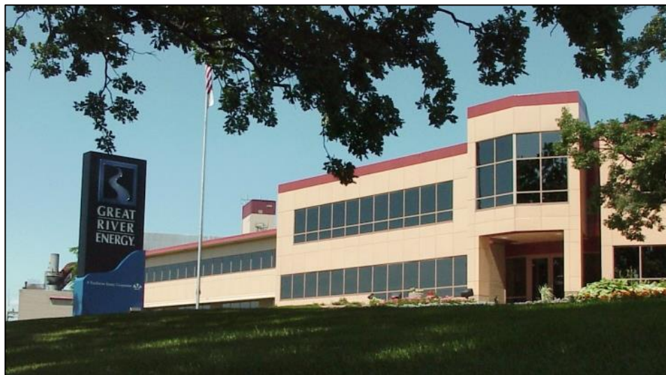
Great River Energy Elk River Campus (Great River Energy)
